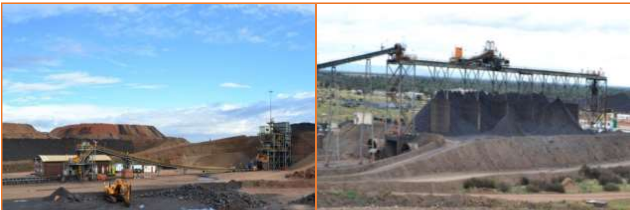
Figures 3 and 4: Tshipi Borwa Manganese Mine processing facilities
