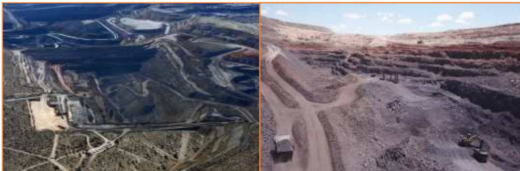
Figures 1 and 2: Tshipi Borwa Manganese Mine Pit
