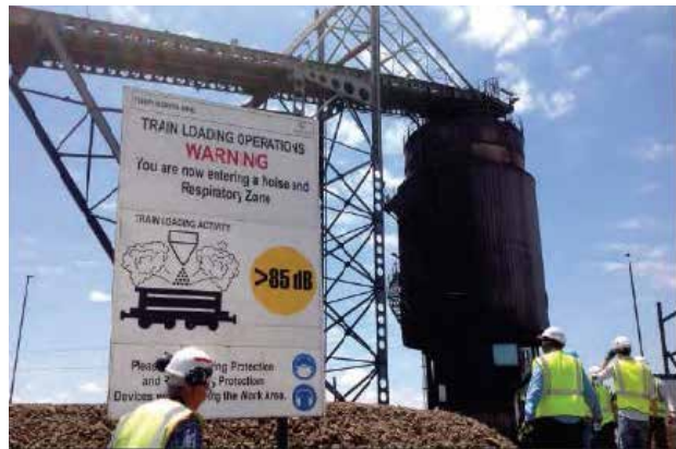
Figure 12: Tshipi mine rapid load out facility
