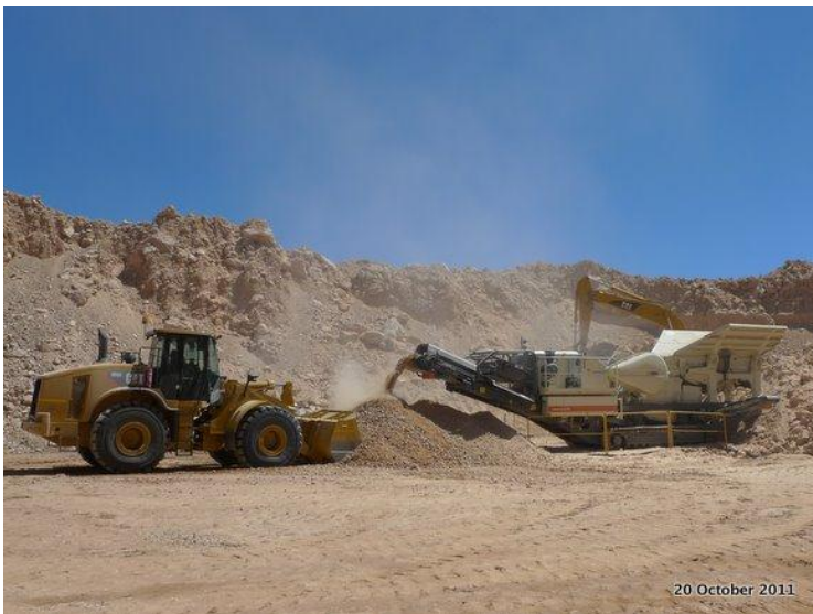
Tshipi Borwa – Waste rock crushing
