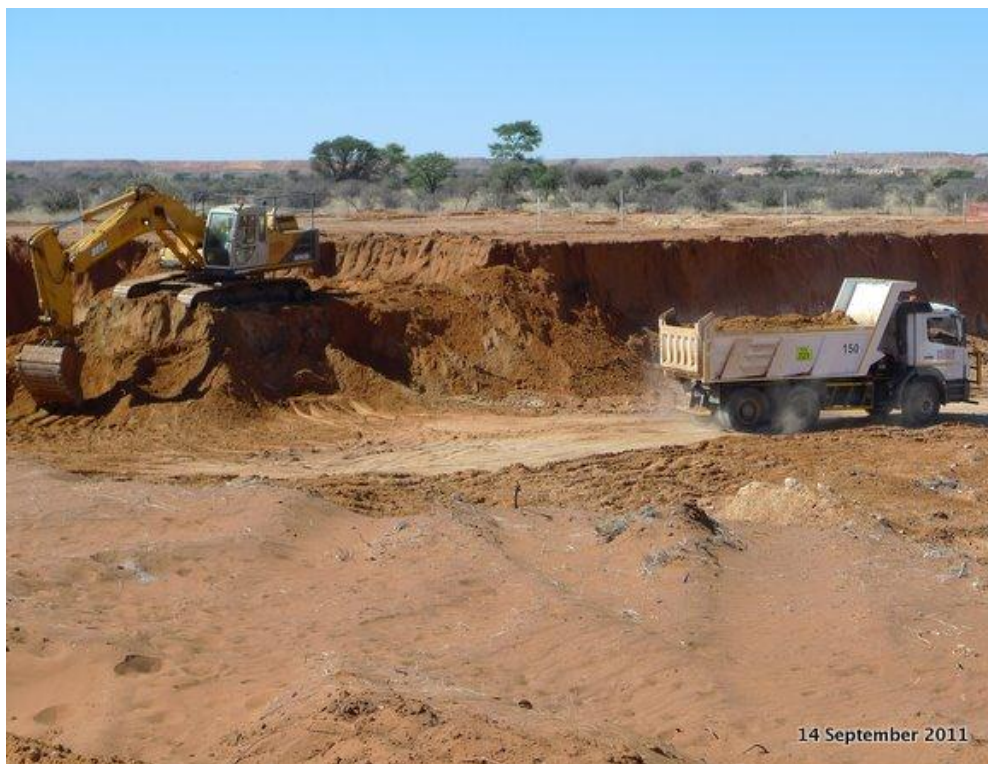
Tshipi Borwa – Storm water pit excavations
