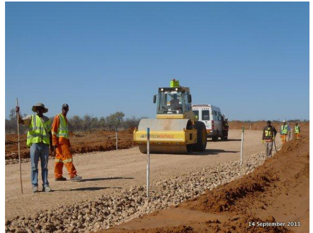
Tshipi Borwa –Railroad siding foundation construction
