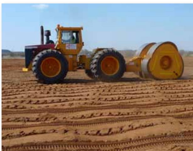
Figure 8 - Impact soil compaction
