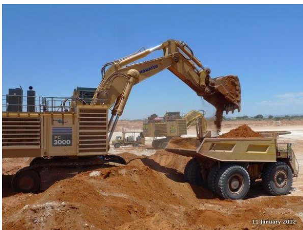
Tshipi Borwa - Mine Pre-stripping underway
