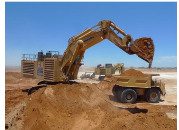
Tshipi Borwa – Open pit overburden removal (13 January 2012)
