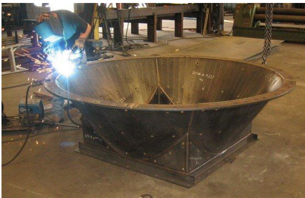
Tshipi Borwa – Rapid load out station under construction
