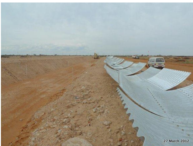
Tshipi Borwa – Stockpile tunnels being assembled
