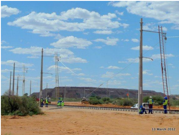
Tshipi Borwa - Overhead traction being installed
