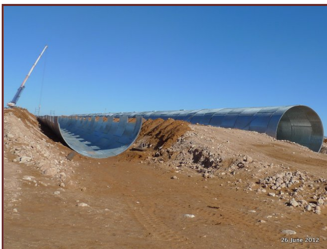
Tshipi Borwa – Stockpile tunnels being assembled
