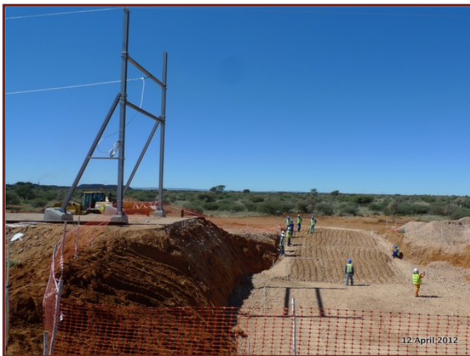
Tshipi Borwa – Rapid load out station under construction
