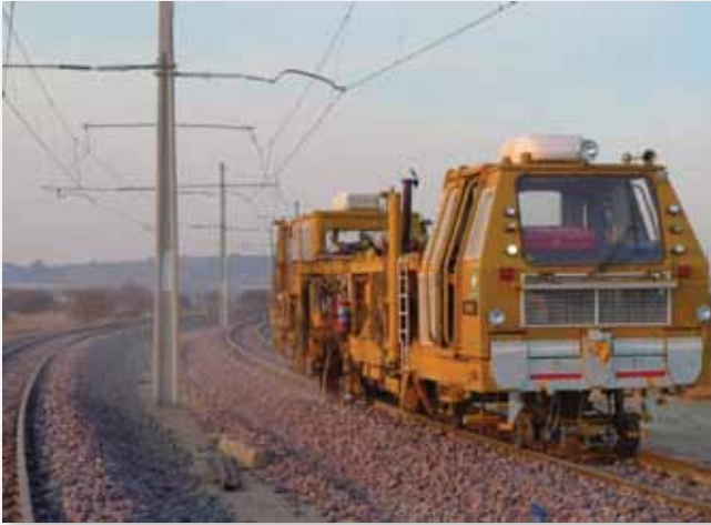
Figure 8. Tshipi Borwa – Rail Tamping
