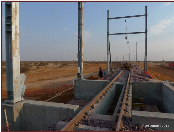
Tshipi Borwa – Load-out station track work complete and vertical columns erected.
