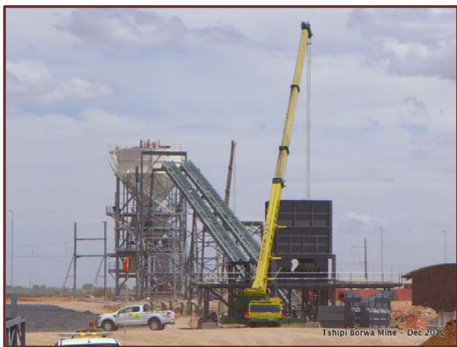
Figure 19 – Tshipi Borwa Construction of the Rapid Load-Out Station and Feeding Conveyors
